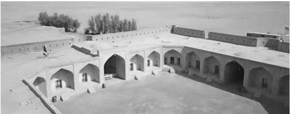
Figure 4: Modern caravanserai. Bigger and more impressive than the one at Bethlehem but illustrates the concept of the raised leewans and a centre courtyard.
